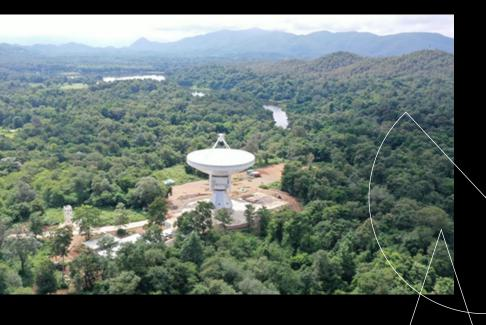
Weight: 450 tons Reflector diameter: 40 m
