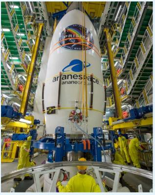
Coupling of the payload fairing around the satellite
