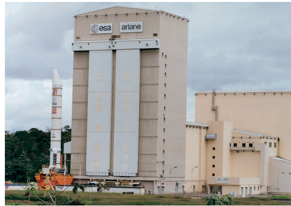
Booster Integration Building (BiP) in Kourou
