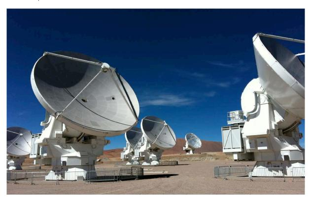
At the center of the observatory is an array of 50 antennas, each with a diameter of 12 meters, operating like a single telescope in the form of an interferometer
