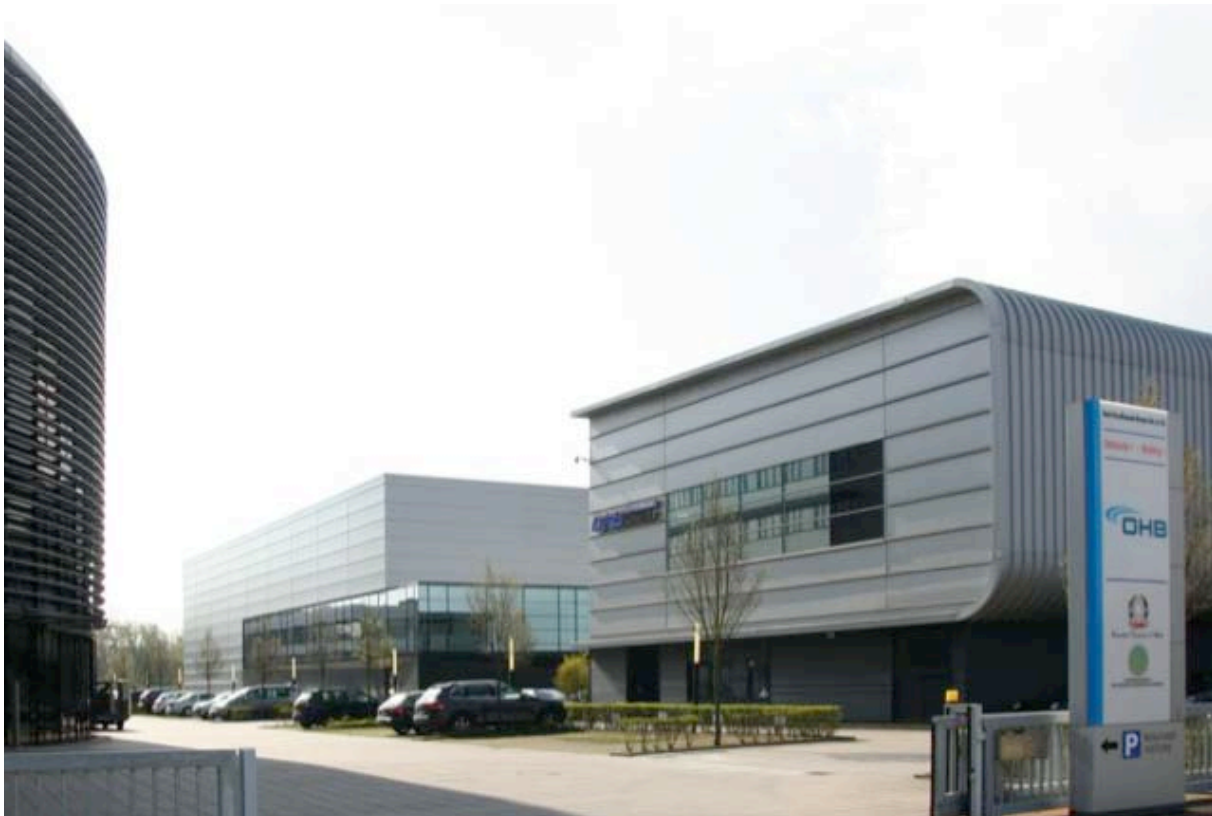
Head office and the new Galileo* integration hall (middle) in Bremen
