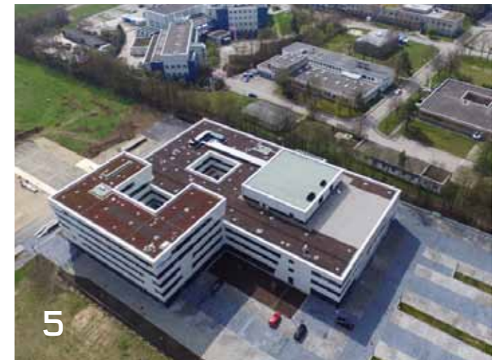
5 Aerial view of the building. Part of the neighbouring DLR Oberpfaffenhofen site can be seen in the background.
