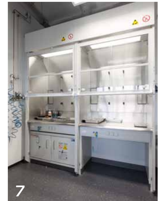
7 Fume cupboards for cleaning printed circuit boards or for bonding and coating work.
